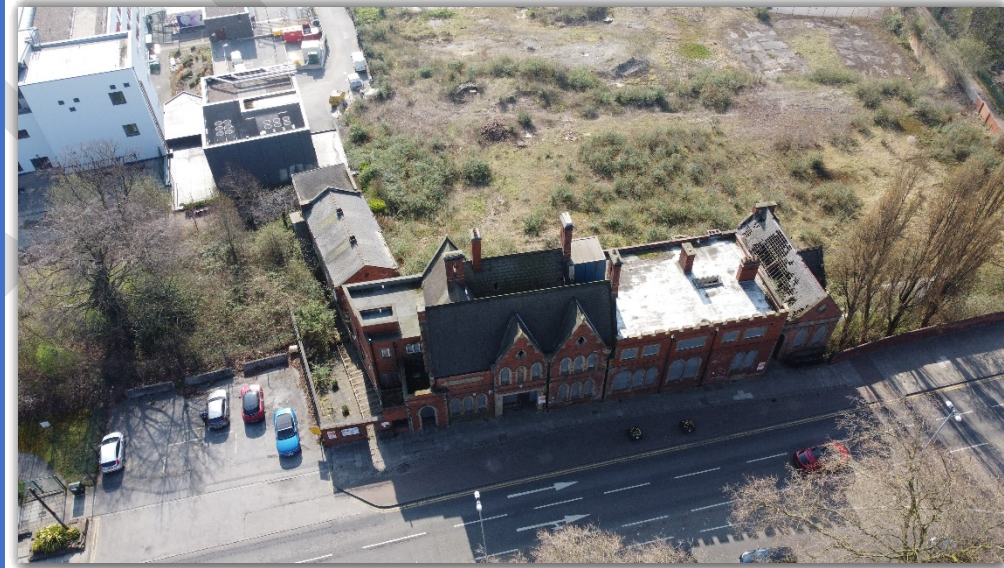
Image: Pontefract Dispensary Building
